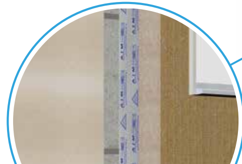
Wall Cavity Barriers completing a vertical compartment line (Full Fill Cavity)
