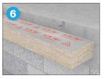
Hold the section of barrier tightly against the abutting section and secure the barrier to the substrate.
